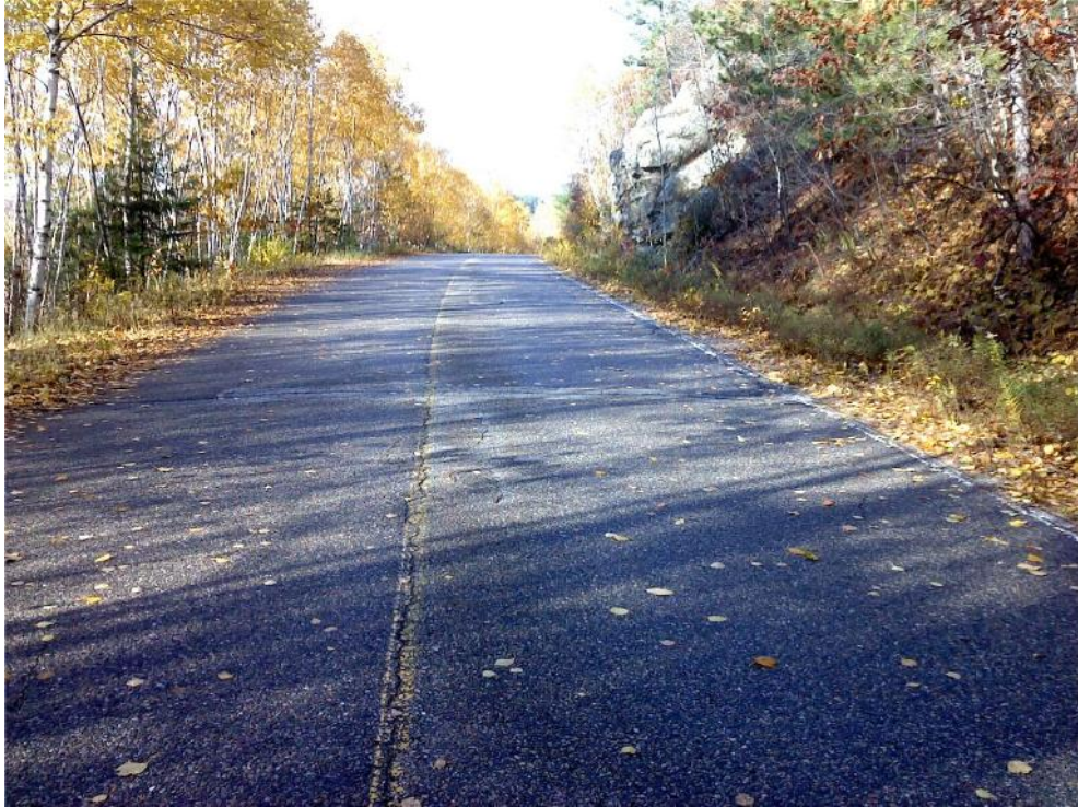
Figure 1: Panel Mine Road in Area 1. Facing West.
