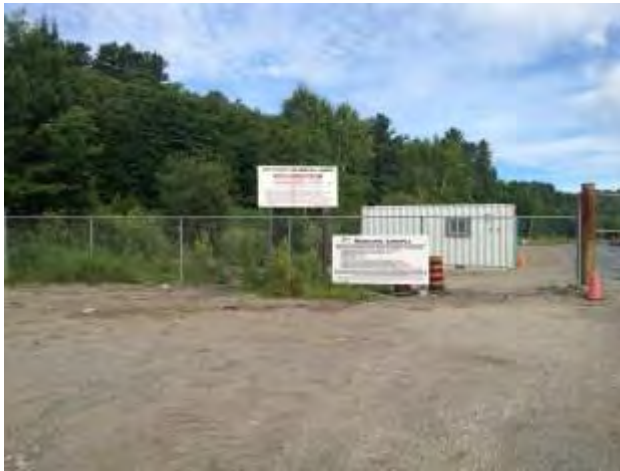
Photo 22: New signs, office space and gate observed during the 2014 field investigation.
